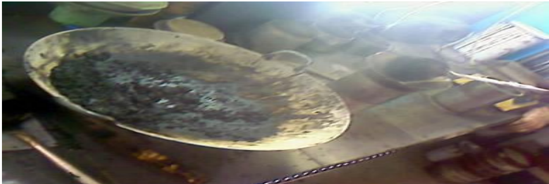
Aggregates and bitumen are mixed together in a pan.
