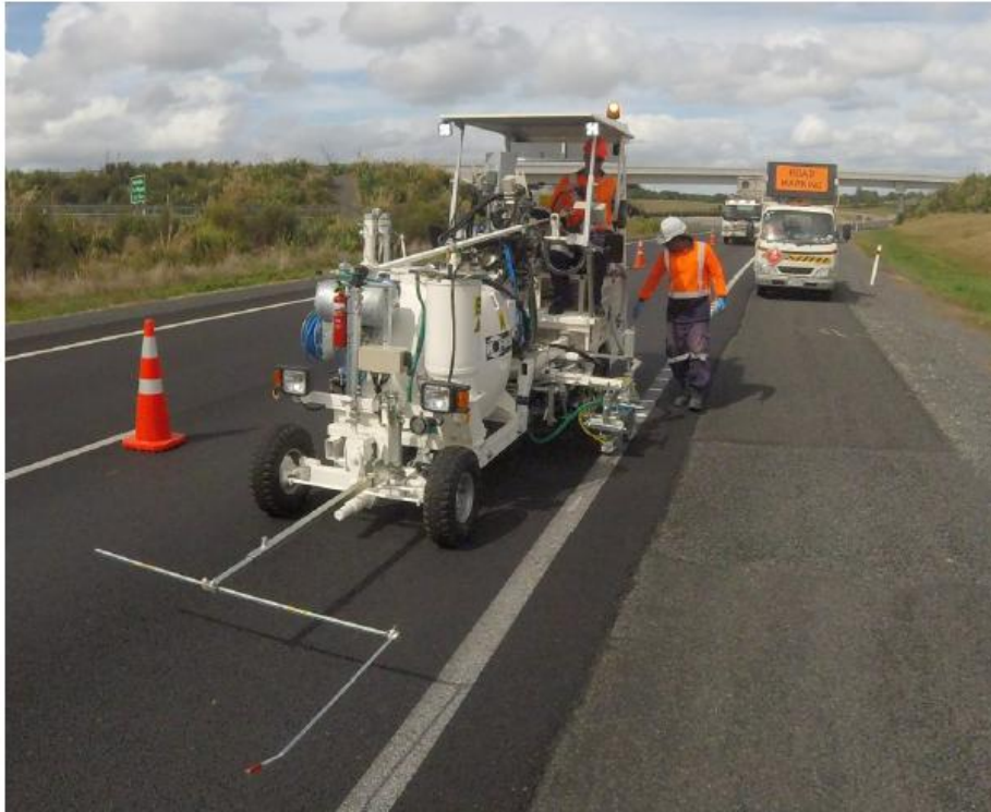
Fig. 5. Installation practice of audio tactile profiled line markings
