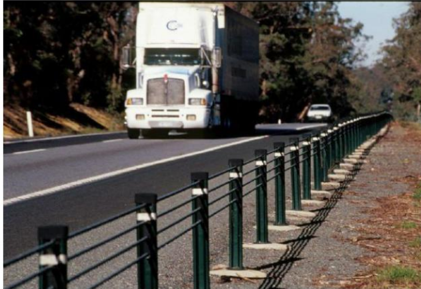
Fig. 3. Wire Rope Safety Barrier
