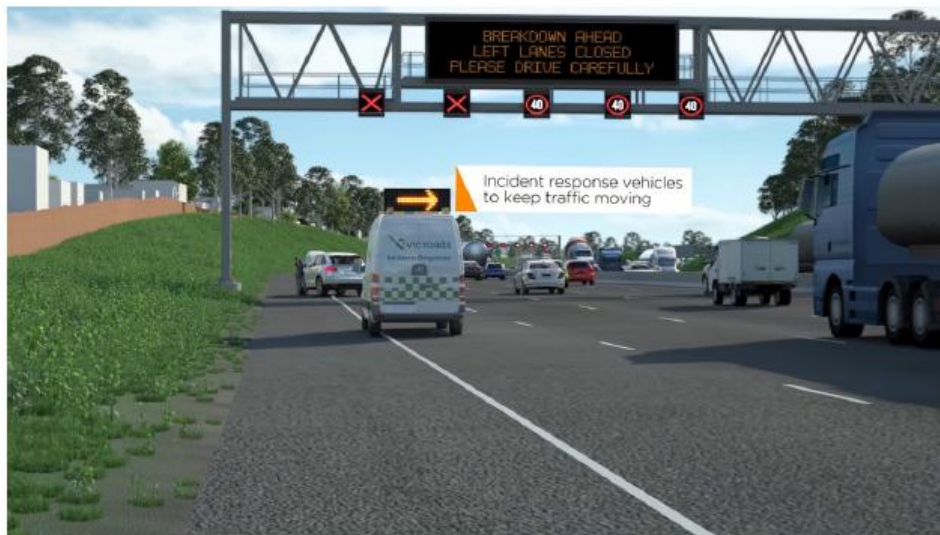
Fig. 6. Monash upgrade freeway management system
